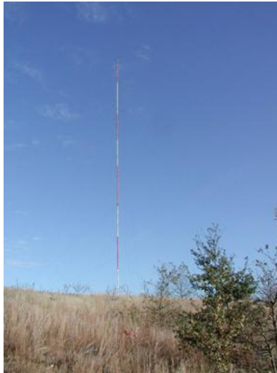
Figure 2 - Monitoring Station/Data Equipment at Thompson Island
