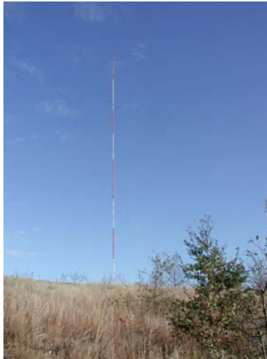
Figure 2 - Monitoring Station/Data Equipment at Thompson Island
