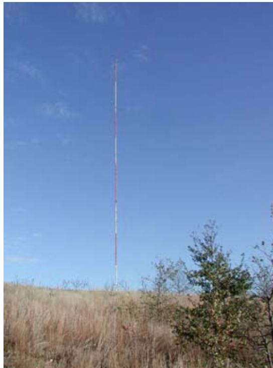
Figure 2 - Monitoring Station/Data Equipment at Thompson Island
