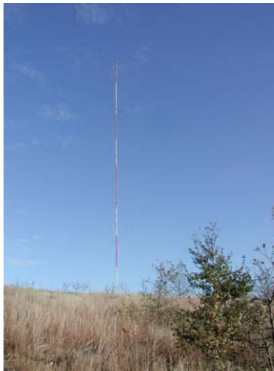
Figure 2 - Monitoring Station/Data Equipment at Thompson Island
