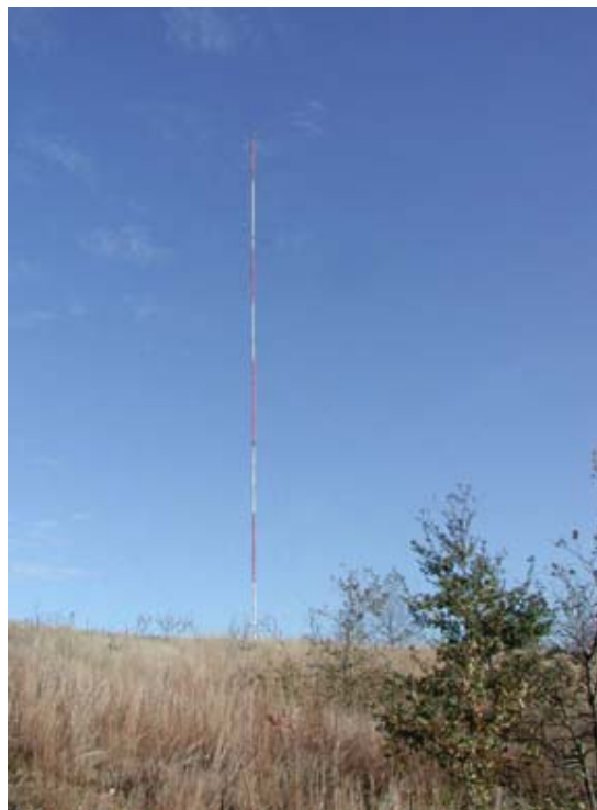
Figure 2 - Monitoring Station/Data Equipment at Thompson Island
