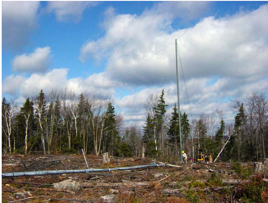
Figure 2 – 50m data tower in Savoy during installation.
