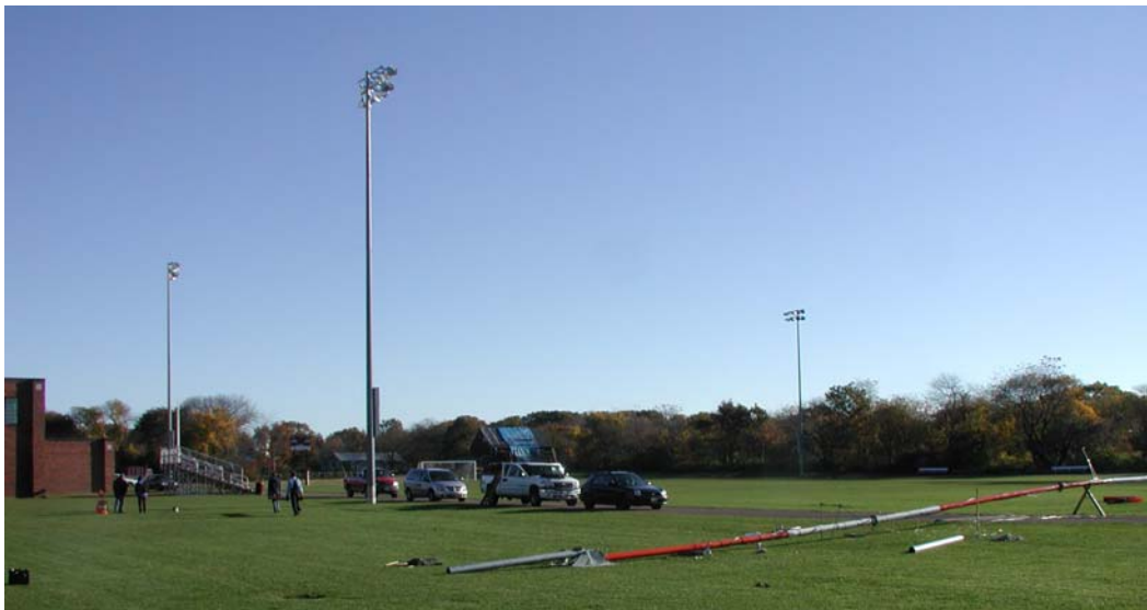
Figure 2 – Preparation to raise the Met-tower at Rockport Site
