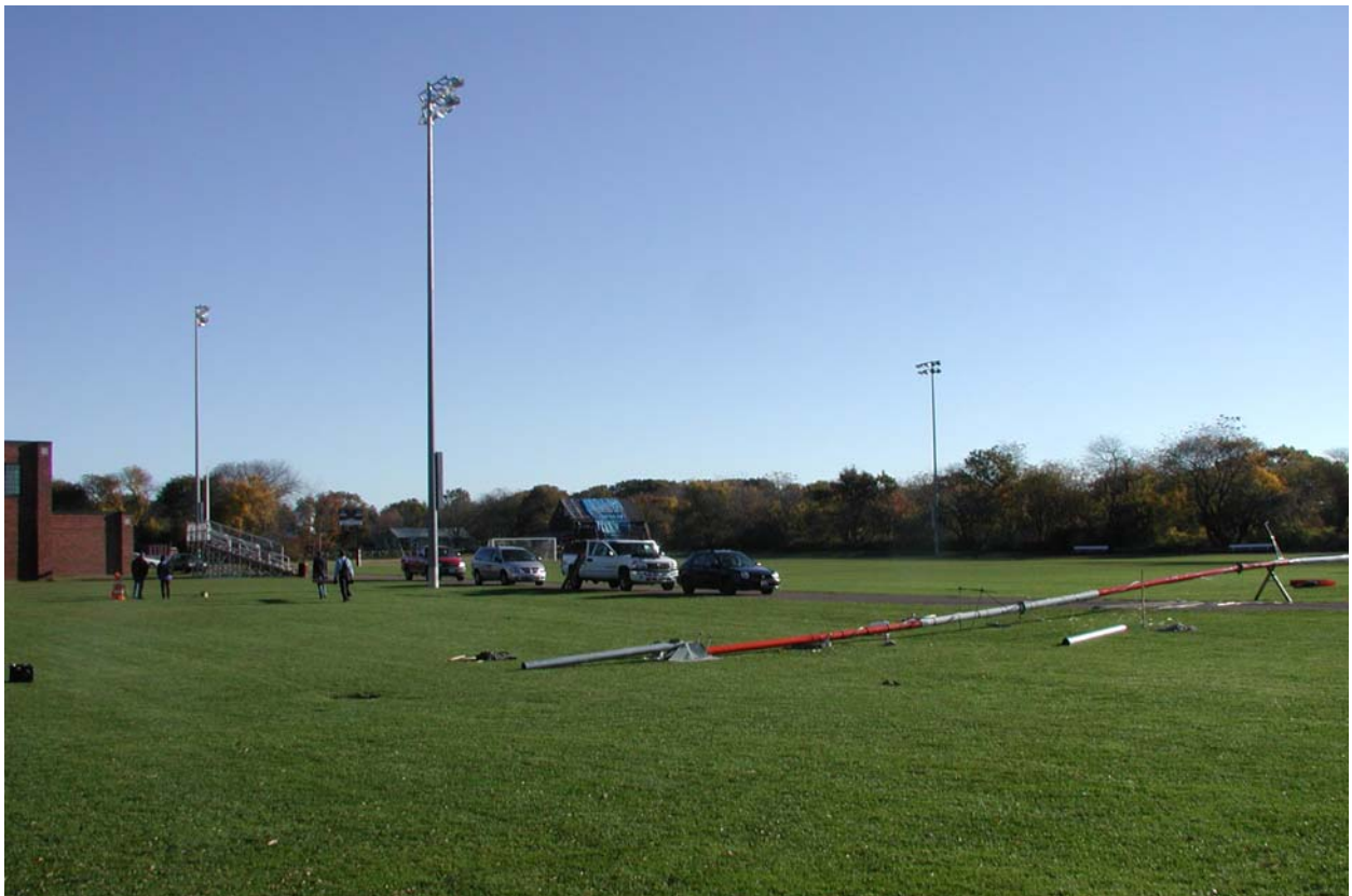
Figure 2 – Preparation to raise the Met-tower at Rockport Site
