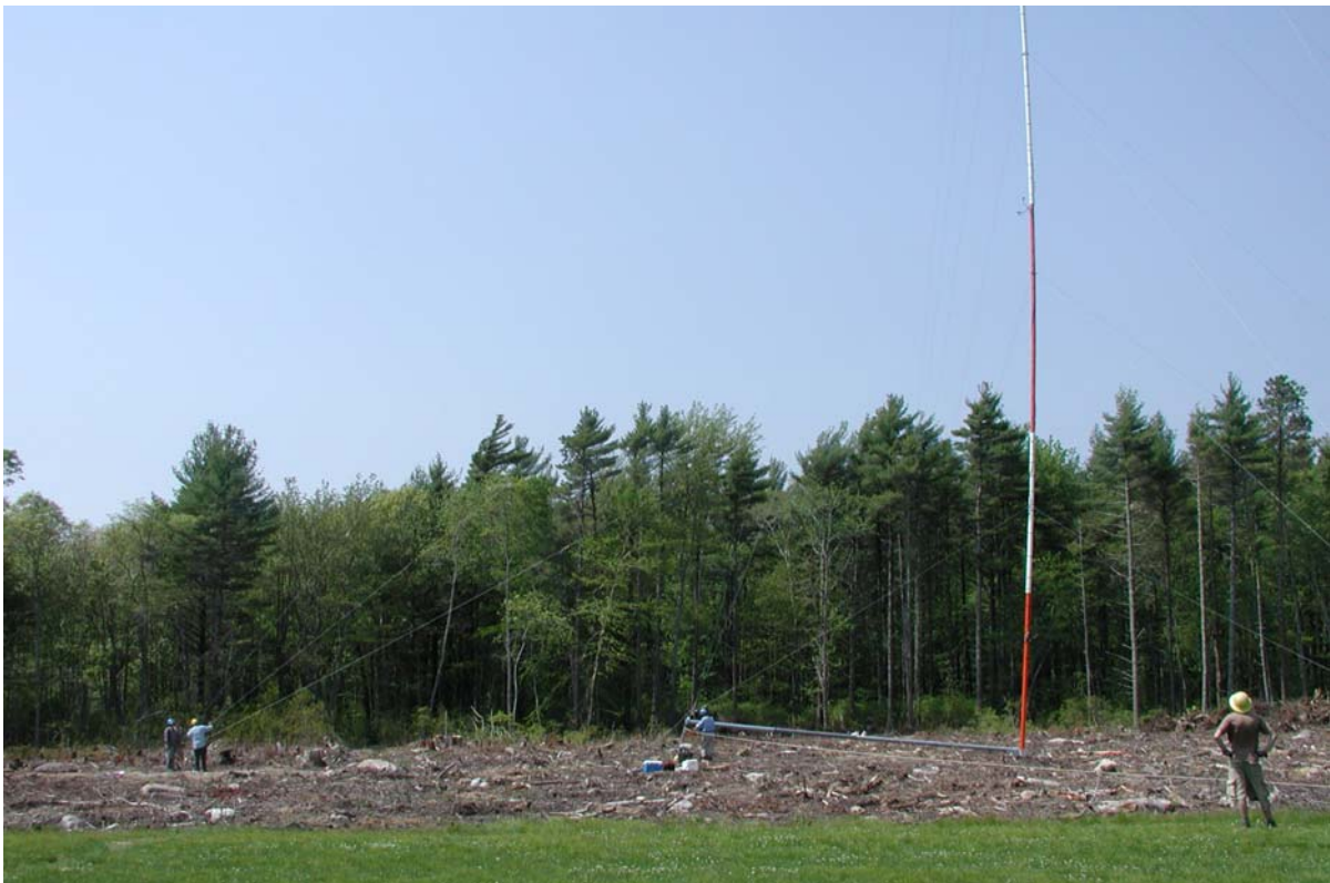
Figure 2 – Raising the Met-tower at ORR Site
