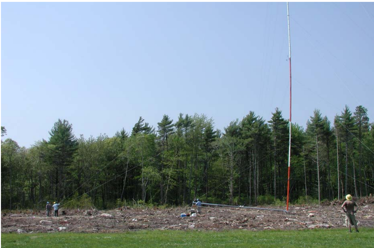
Figure 2 – Raising the Met-tower at ORR Site
