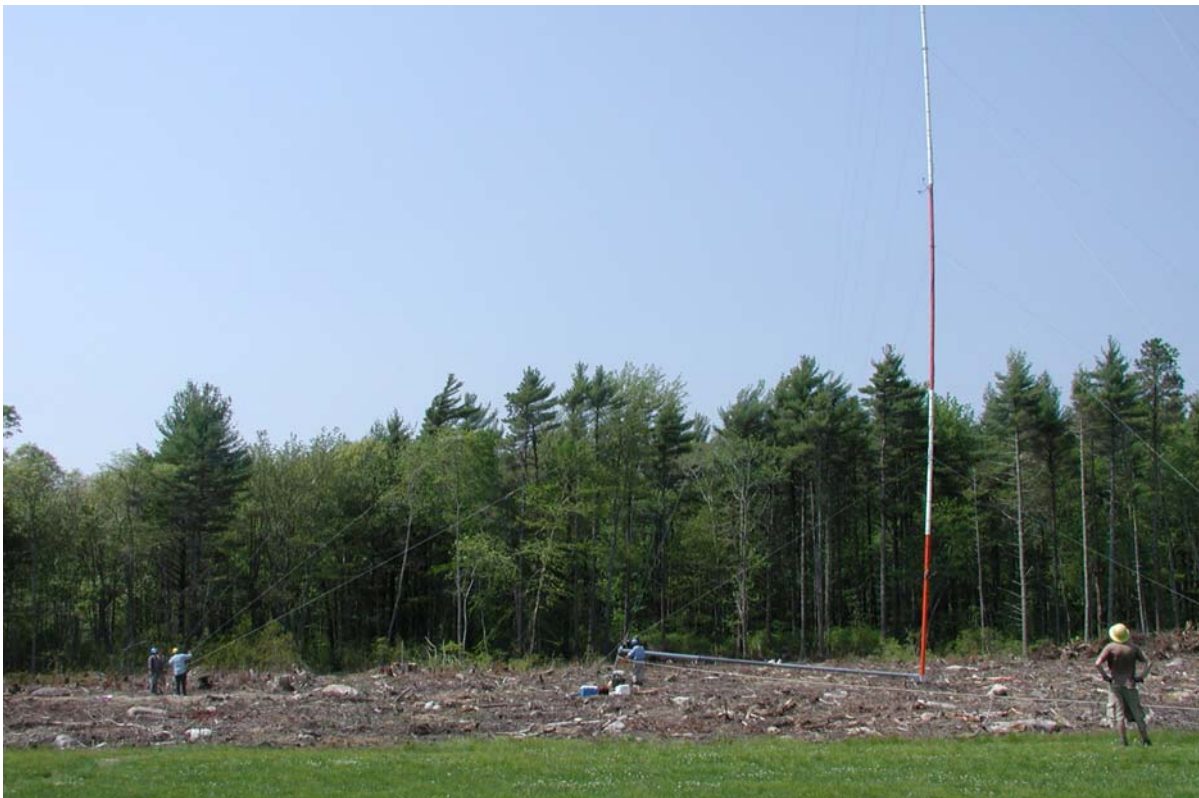
Figure 2 – Raising the Met-tower at ORR Site
