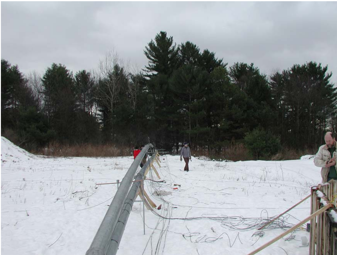
Figure 2 Preparation to Raise Met-tower at Narragansett Site
