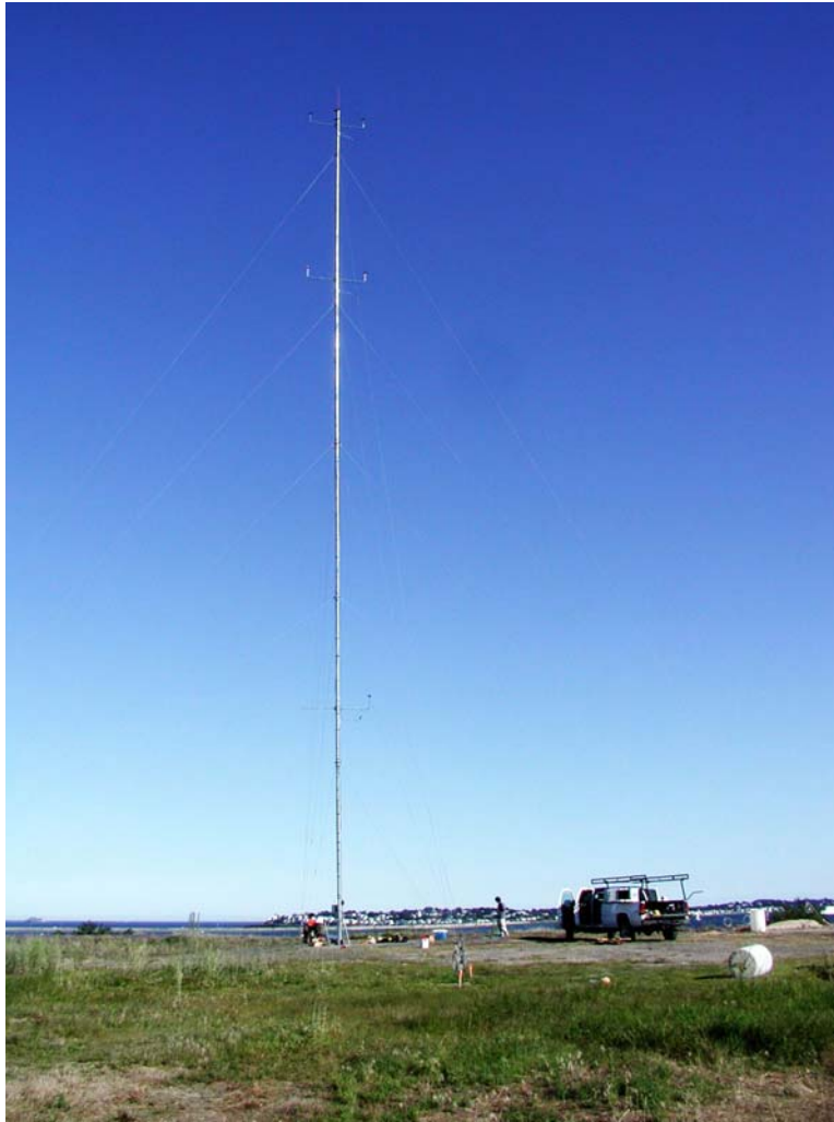
Figure 2 – Lynn monitoring tower. Booms and anemometers are at 10, 30, and 39 m.
