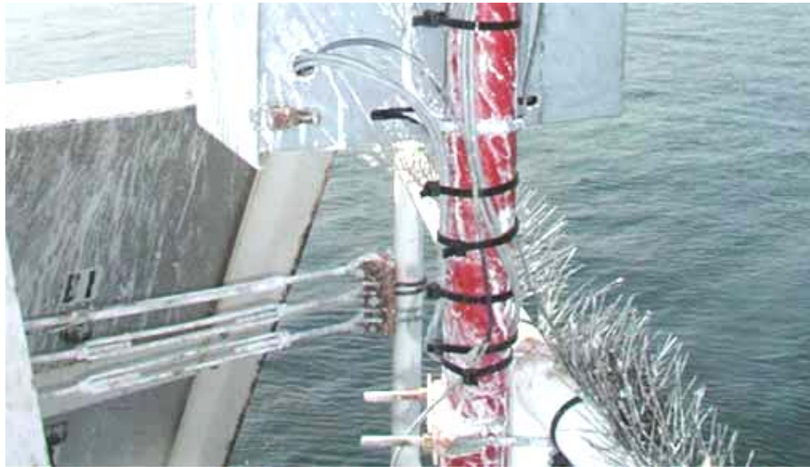
Figure 3 - Railing stiffener connecting PV bracket to rail
