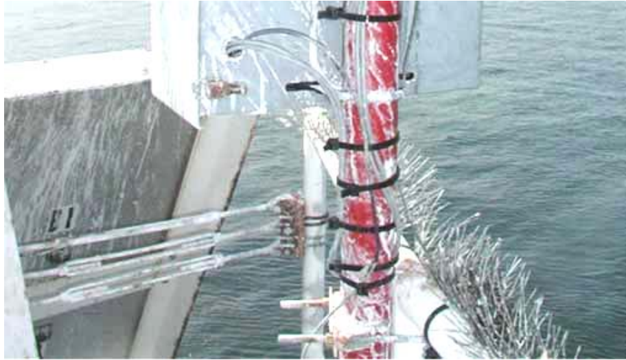
Figure 3 - Railing stiffener connecting PV bracket to rail
