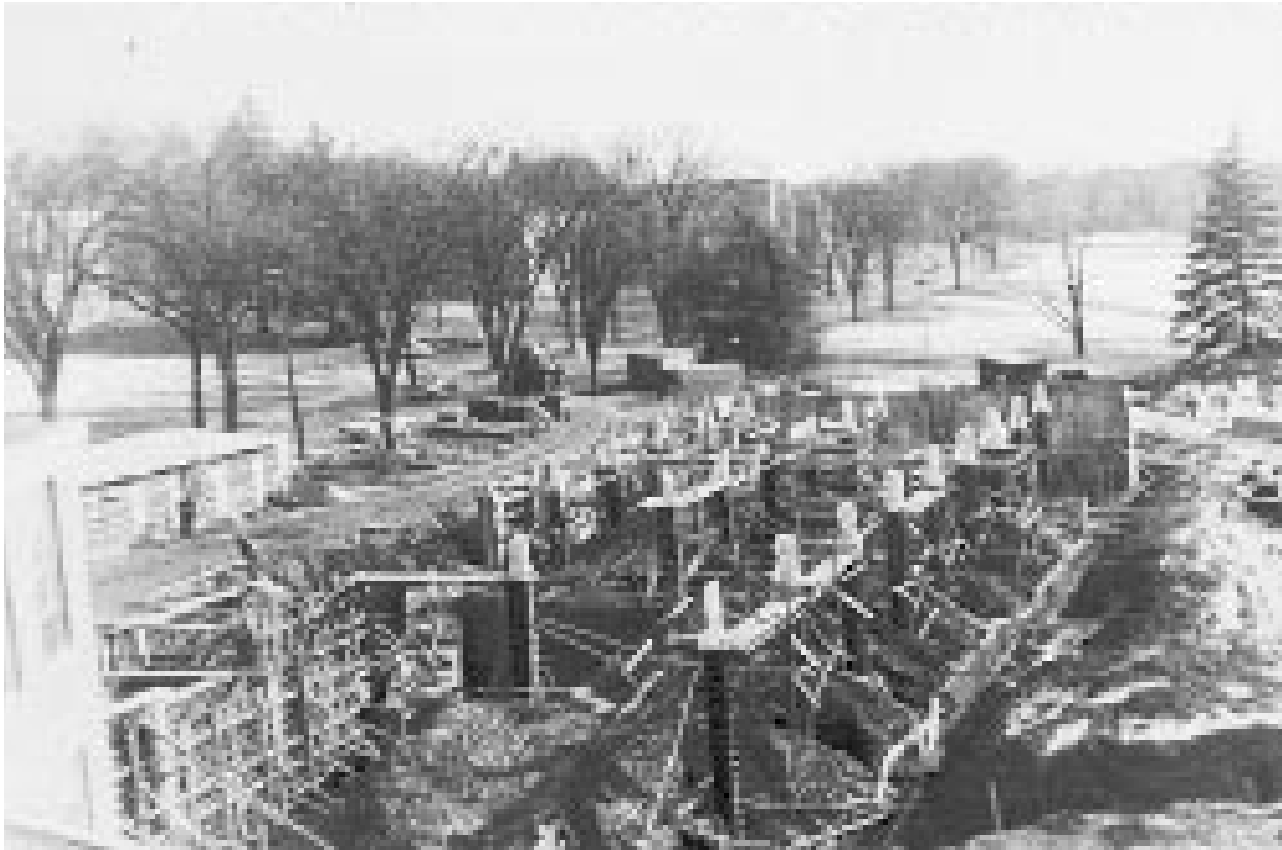
Construction of the Hasbrouck Addition, ~1962
