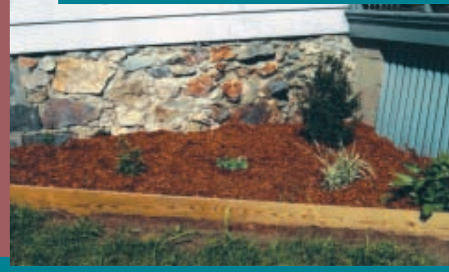
Top: Before—bare soil in drip zone (1660 ppm). Bottom: After—mulched planting bed covering soil.
