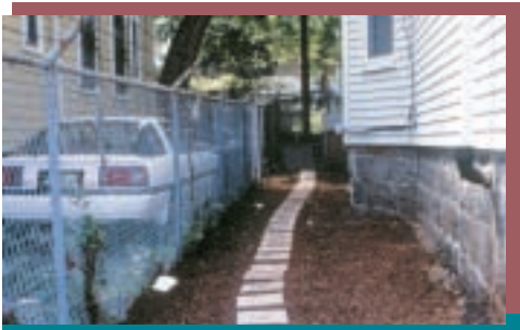
Install stepping stones to prevent contaminated soil from being tracked into the house.
