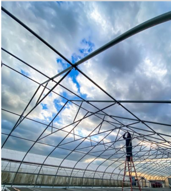
High tunnel reconstruction underway at Four Town Farm in Seekonk, MA after snow and wind collapsed the tunnel a few weeks ago. Photo: Four Town Farm
