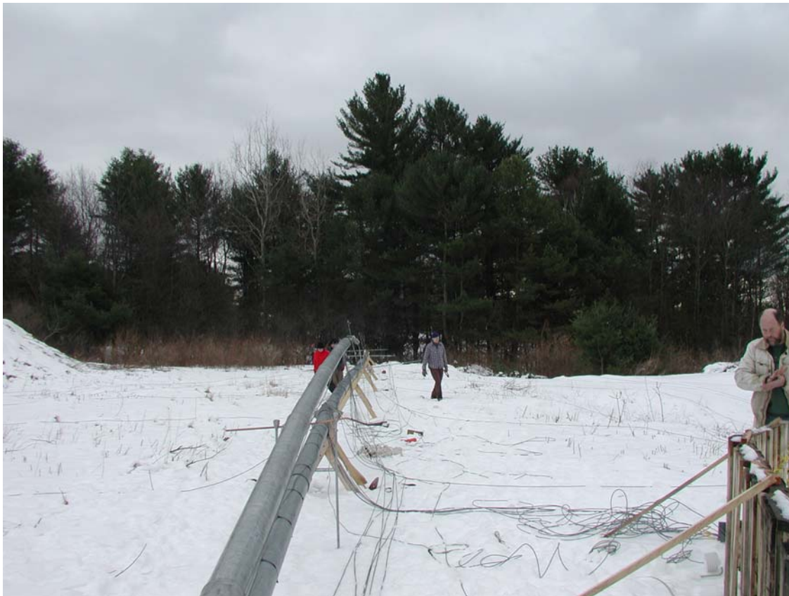
Figure 2 – Preparation to Raise Met-tower at Narragansett Site
