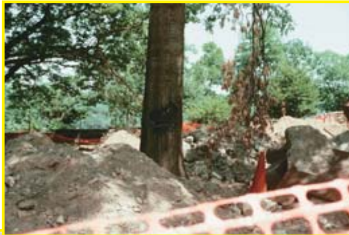
Although the root zone of this tree was defined with snow fencing, lack of adequate site supervision made that a wasted effort (left). The broken limb and damaged bark on the tree above are the most visible injuries, but the excavated material piled beneath it will soon suffocate the roots.
