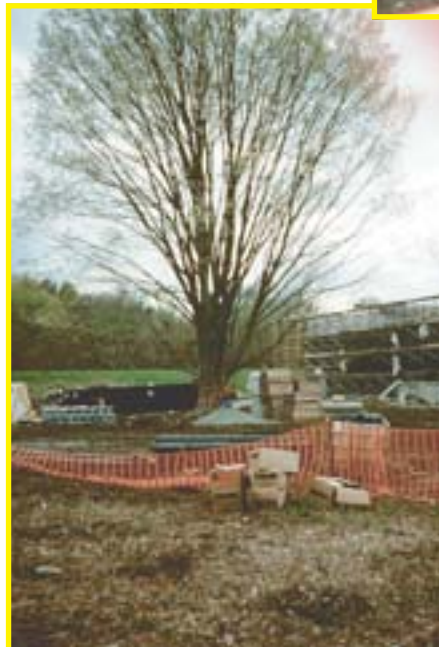
Although the root zone of this tree was defined with snow fencing, lack of adequate site supervision made that a wasted effort (left). The broken limb and damaged bark on the tree above are the most visible injuries, but the excavated material piled beneath it will soon suffocate the roots.
