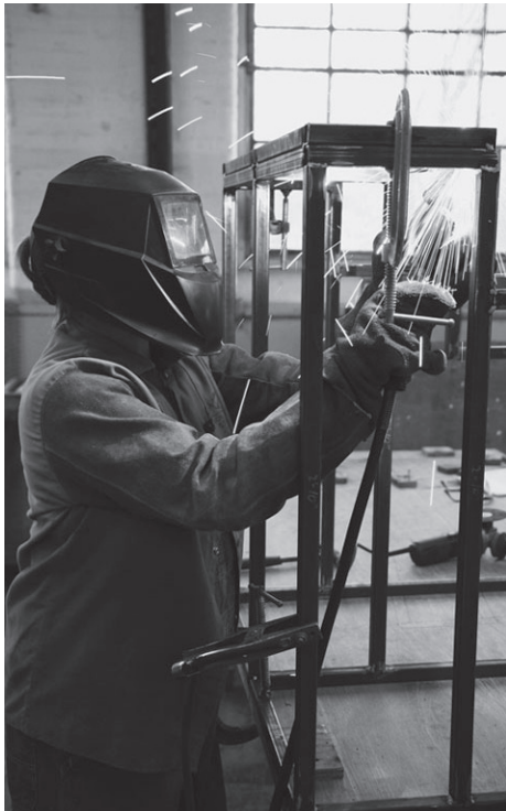
Davis welding steel stairs for The Boston Conservatory's production of Follies in Boston.
