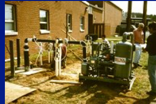
Example of Active Venting System
