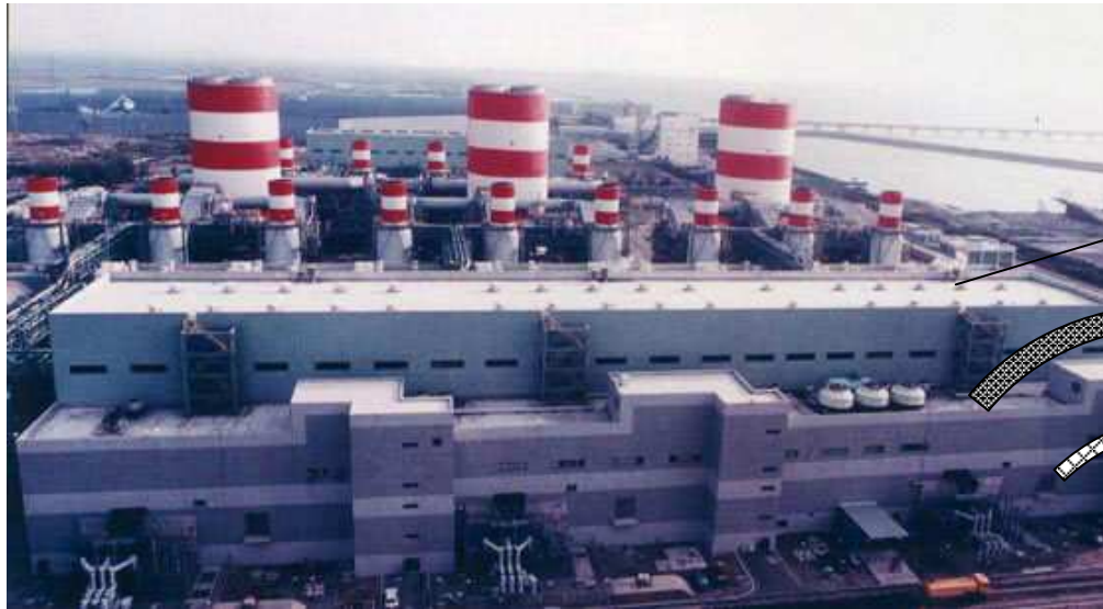
Natural gas power generating plant
