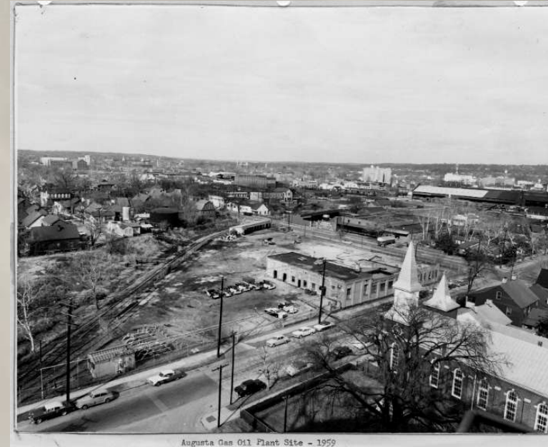
Augusta Gas Oil Plant Site - 1959
